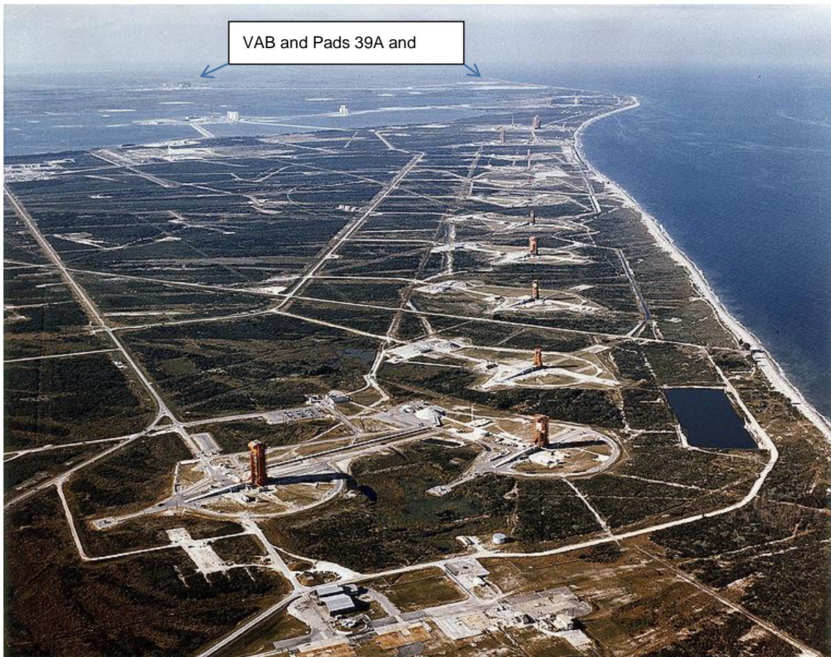
Figure 28. Cape Canaveral Air Force Station and Missile Row. The view is looking north, with the NASA Vehicle Assembly Building (VAB), Crawlerway, and Pads 39A and B under construction, in the top of the 1964 NASA photo.
